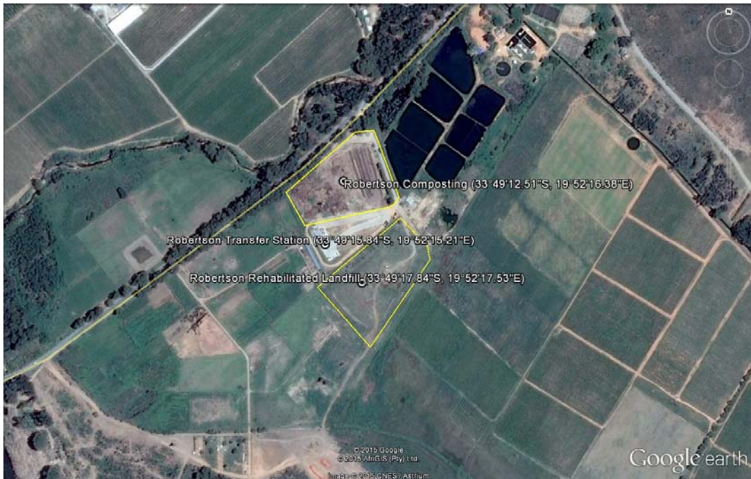
Figure 3-27: Robertson Transfer Station
