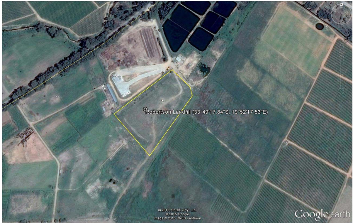
Figure 3-20: Robertson Rehabilitated Landfill
