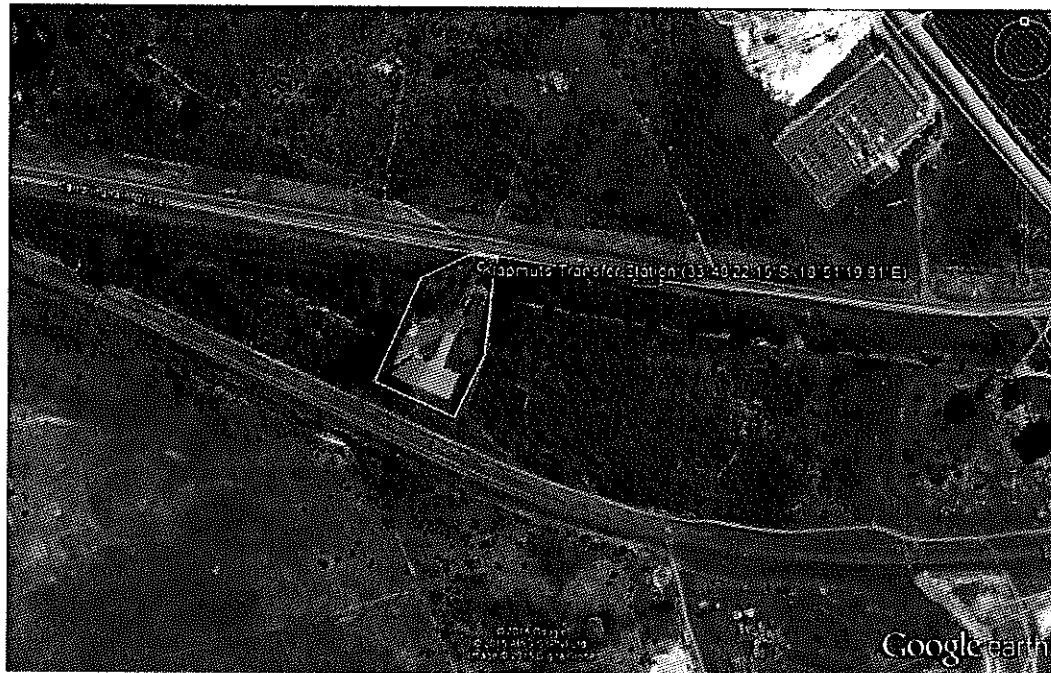
Figure 3-30: Klappmuts Transfer Station
