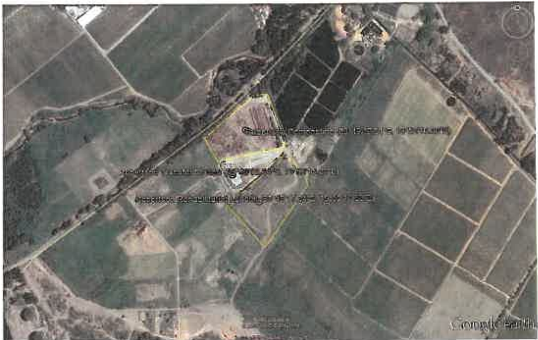
Figure 3-27: Robertson Transfer Station
